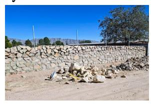
Repair and reinforcement work on the rockwall at the southeast corner of the pond lot, which had fallen in September is nearing completion.
